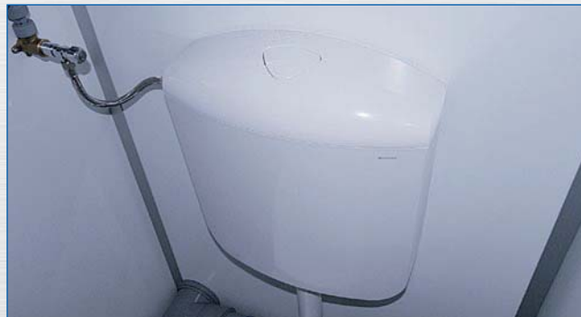
Flushing cistern with water saving device
