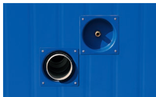
Water connection, embedded in the wall
